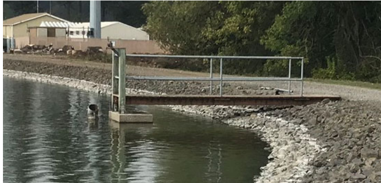
Figure 4-9 | Typical Lagoon Outlet Structure
