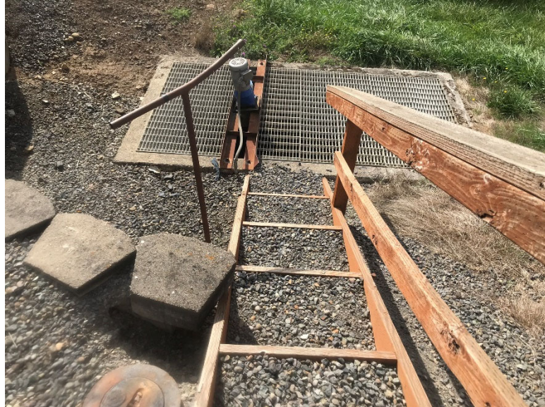
Figure 4-10 | Chlorine Contact Chamber Inlet Structure
