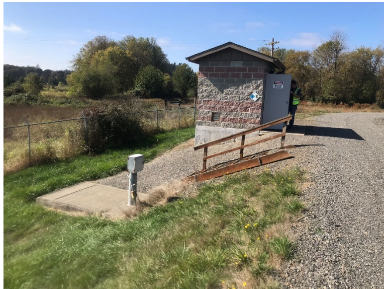
Figure 4-11 | Chlorine Contact Chamber Outlet and Dechlorination Building
