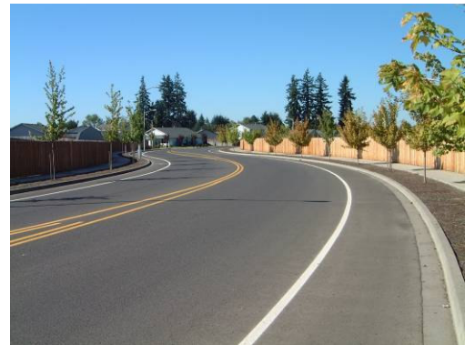
Suburban collector road through residential area with bike lanes, landscaping and sidewalks.
